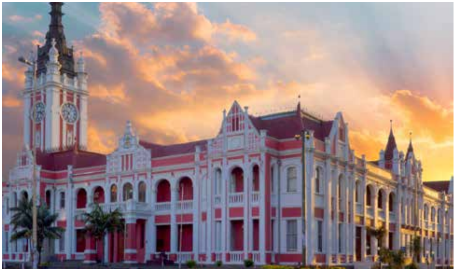
Buffalo City Municipality Building, East London.
